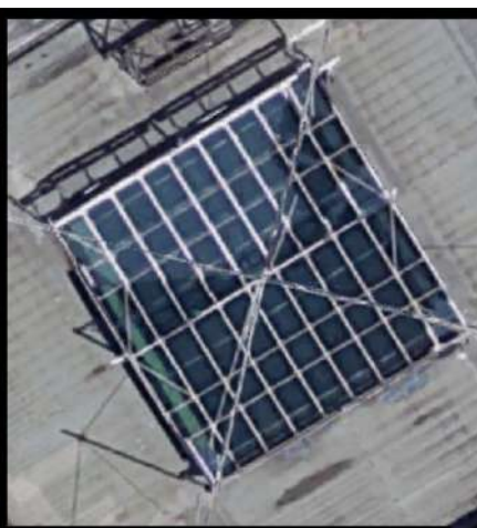
Skylight Google Earth 2019
