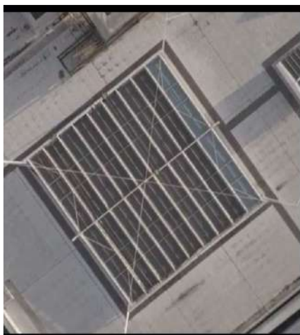
Skylight in early June 2017
